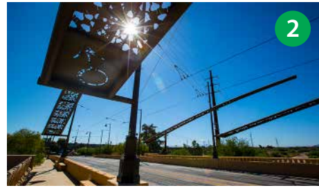
2 Luis G. Gutierrez Bridge Structural Grace Inc., 2014 Cushing Street
