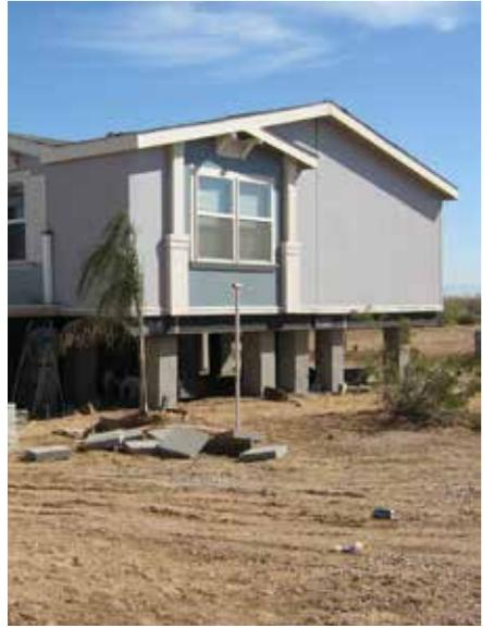
*An elevated manufactured home on a flood resistant foundation.*
