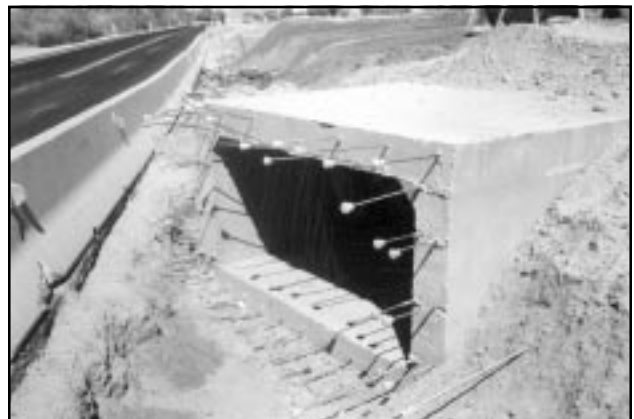
Work underway on Avra Valley Road Extension Improvements
