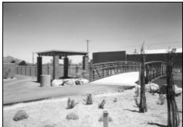
Tucson Diversion Channel River Park Improvements
